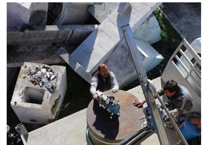
Above: The existing 1960s wastewater treatment plant, was modified and structures cut and reused. https://landezine.com/transforming-the-aproz-wastewater-treatment-system-into-a-playground-by-en-dehors/
