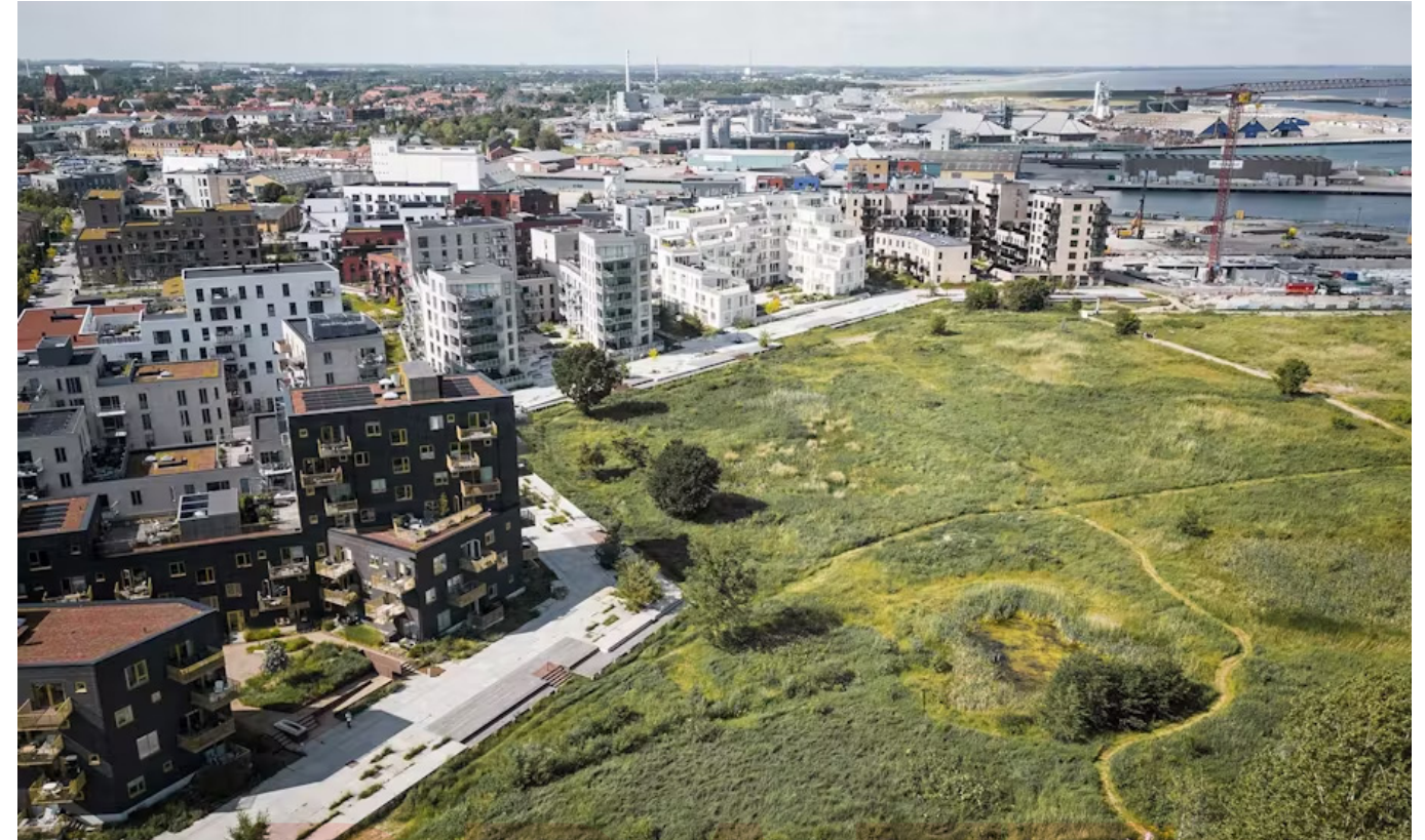
Above: View of the promenade and interface to the adjoining salt meadow. The promenade provides flood protection for the development. Source: https://www.archdaily.com/996753/the-south-harbor-of-koge-sla
